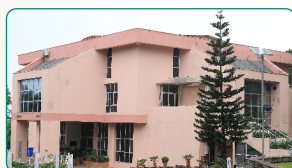
Library and Auditorium
